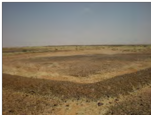
Example of a Newly Built Stone Bund or Banquette in Niger
